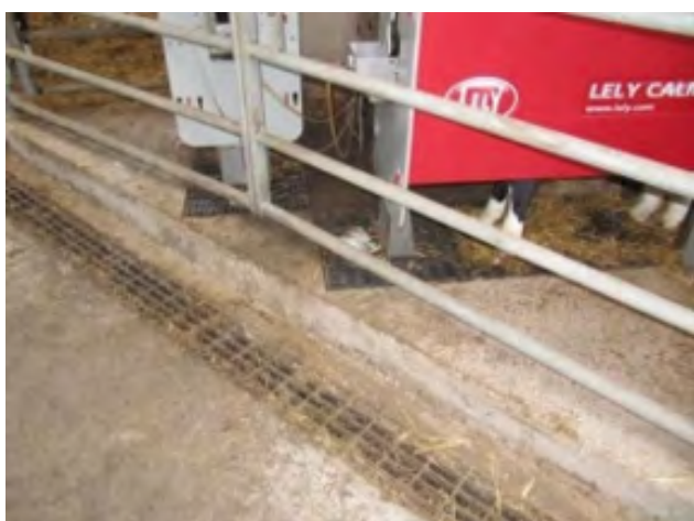
Figure 24: Well designed drainage for automatic feeders will maintain cleanliness
