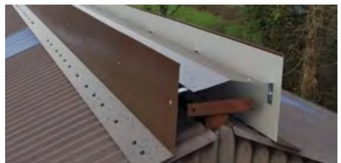
Figure 14: Outlets above eave height are required to release stale air
