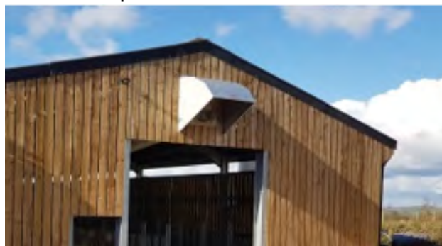
Figure 18: Fan and Outlet of a PPTV system
