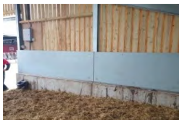
Figure 8: Plastic wall coatings to reduce cleaning time and bacterial load
