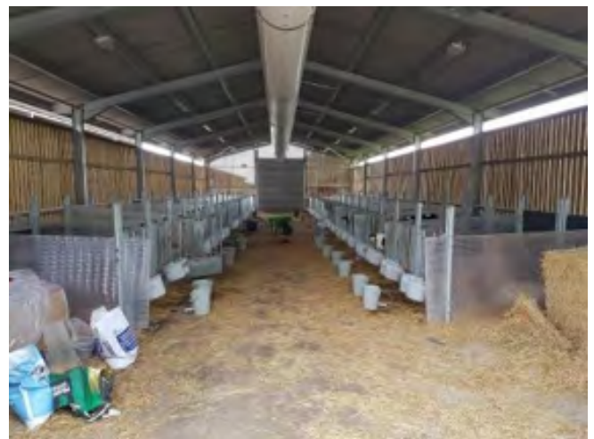
Figure 13: Well designed calf house with ventilation system
