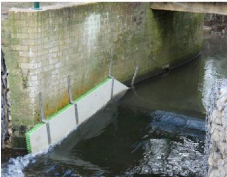
Figure 4.13: Installed pass, showing brackets and fixings
